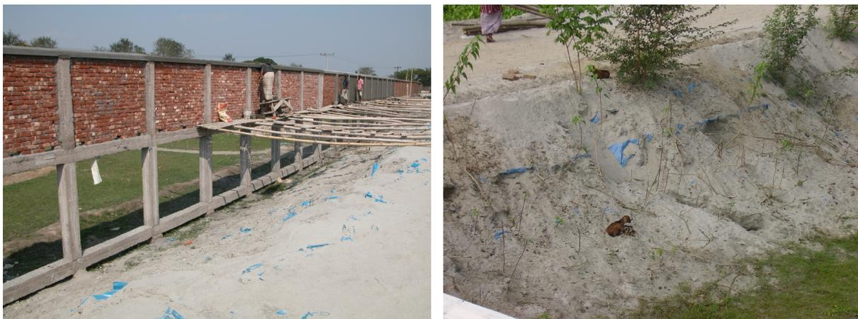
**Figure 18** Base foundations in Bangladesh, here at the Titas hospital complex and its access road, consist of alternating layers of sandy material and plastic sheeting (the left picture showing the wall around the hospital complex, was photographed by B. Planer-Friedrich in February '07, the right one shows the access road to the hospital, taken by the author in November '07)
